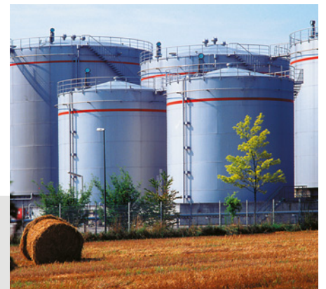
Industrial steel constructions
